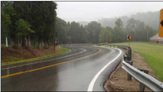
Deficient geometric features are adjacent to Highland-Turner Elementary School.
